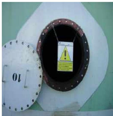
Figure nº 2. Access to the inside of the tank.
