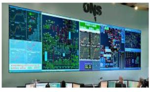
Figure 1.Typical Installation of a Room of the Electrical Power Control and Operation System (source: ONS, 2014).
